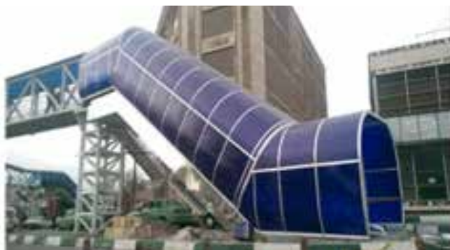
Figure 2: Utilizing Escalator for Mechanized Pedestrian Bridges in Tehran
