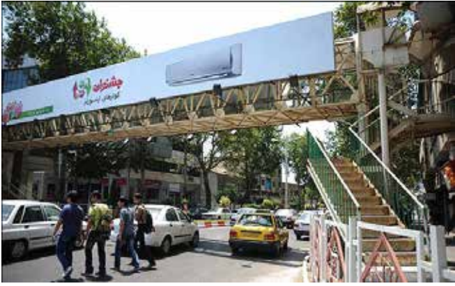
Figure 1: Low Functional Efficiency of Pedestrian Bridges in Tehran
