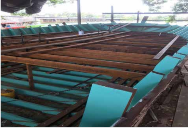
Figure 18: Pelekun that has been Installed
