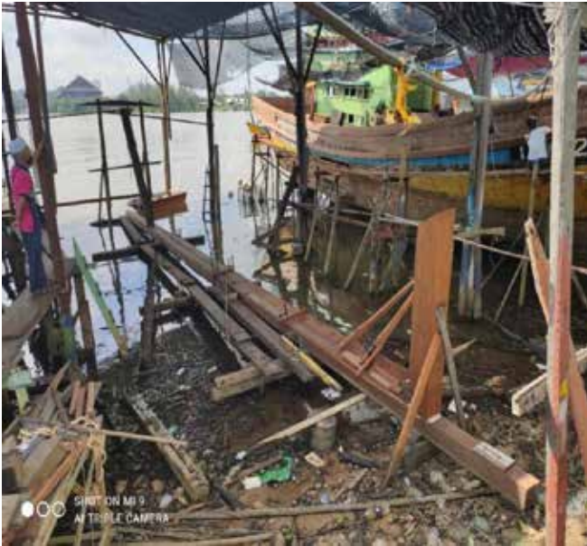
Figure 5: Keel and Stem Installed by Boatbuilder
