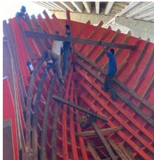
Figure 17: Setel that has been Installed on the Boat Wall
