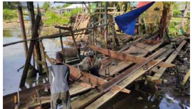
Figure 12: Installation of Belly Kun
