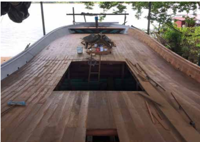
Figure 19: Floorboards are being Installed
