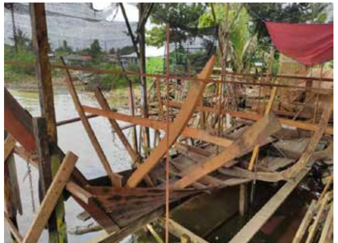
Figure 13: Installation of Title Kun
