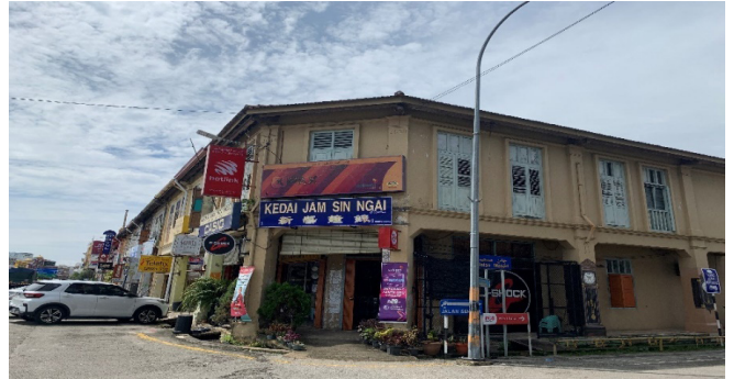
Photo 6: Obvious damage to row of window panels on Jalan Sulaimani shophouses
