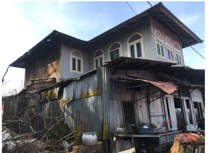
Photo 7: Rear View of Building K52
