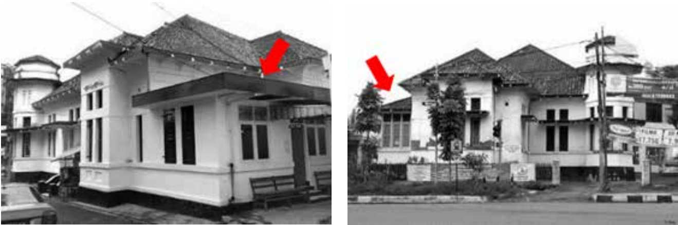
Figure 5: The additional room blocks the entry of air and sunlight (source: Author, 2024)
